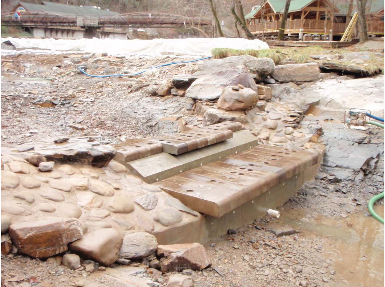
Figure 6 Adjustable precast whitewater features recently installed at an MWDG project in North Carolina.
