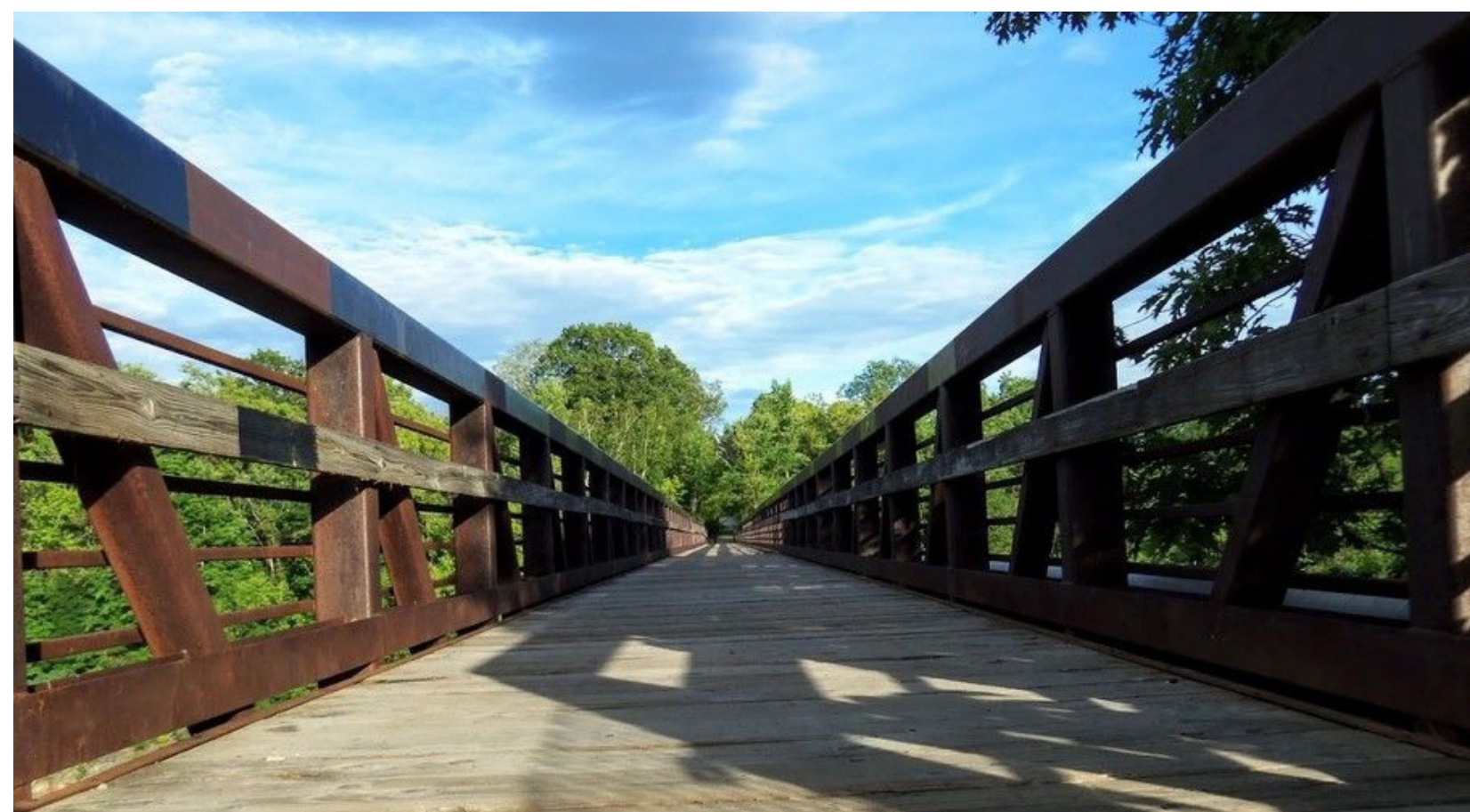
EXISTING PEDESTRIAN BRIDGE
