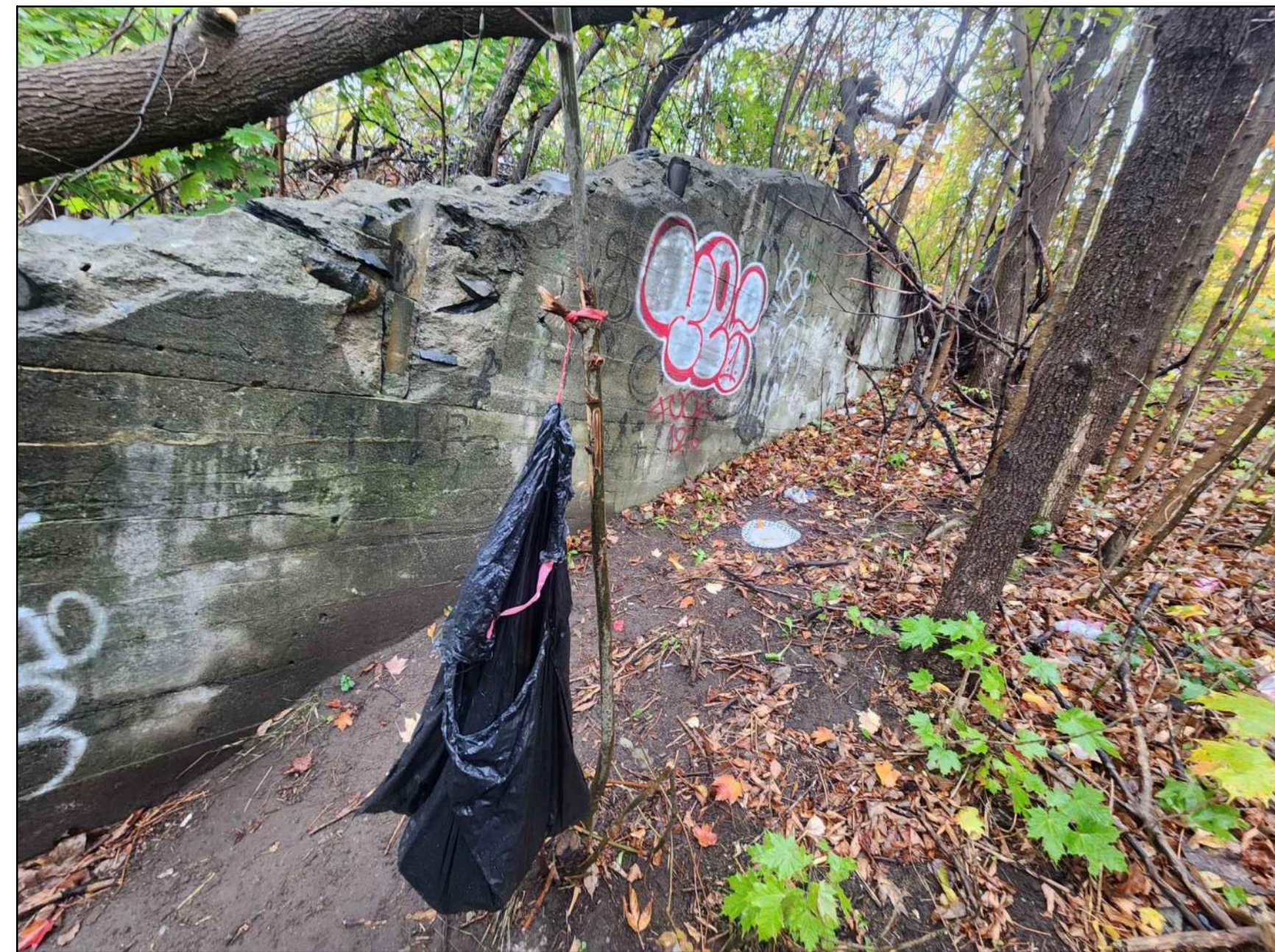
DEMOLITION AREA 1 PHOTO 1 - EXISTING FOUNDATION WALL
