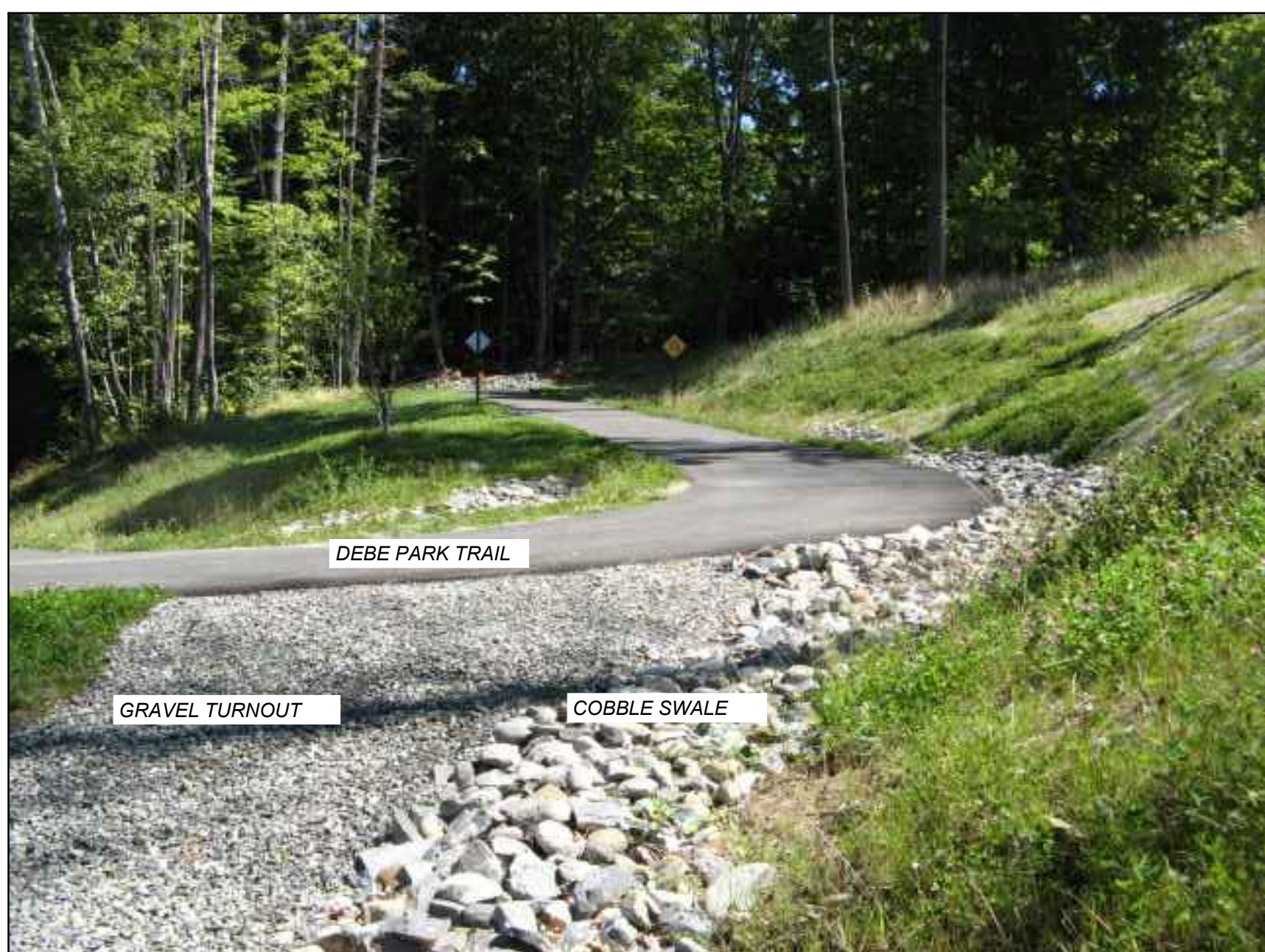
DEMOLITION AREA 2 PHOTO 2 - EXISTING GRAVEL TURNOUT AND COBBLE SWALE
